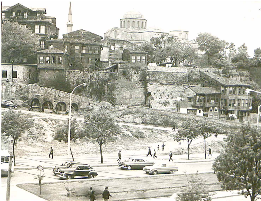
Figure 2. Zeyrek district with wooden houses with bay windows Source: Istanbul Metropolitan Municipality, 2006.
