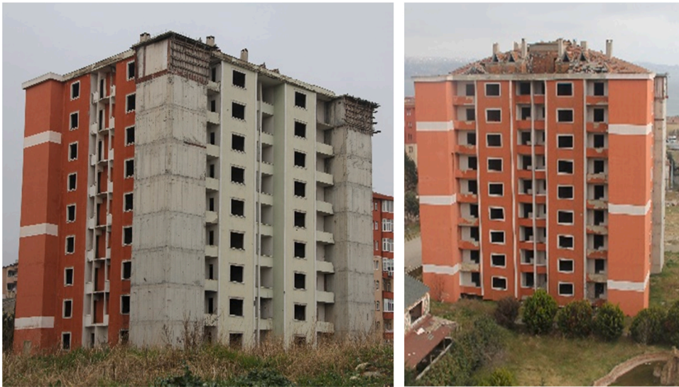
Fig. 6. Overview of Building C (retrofitted with shear walls).
