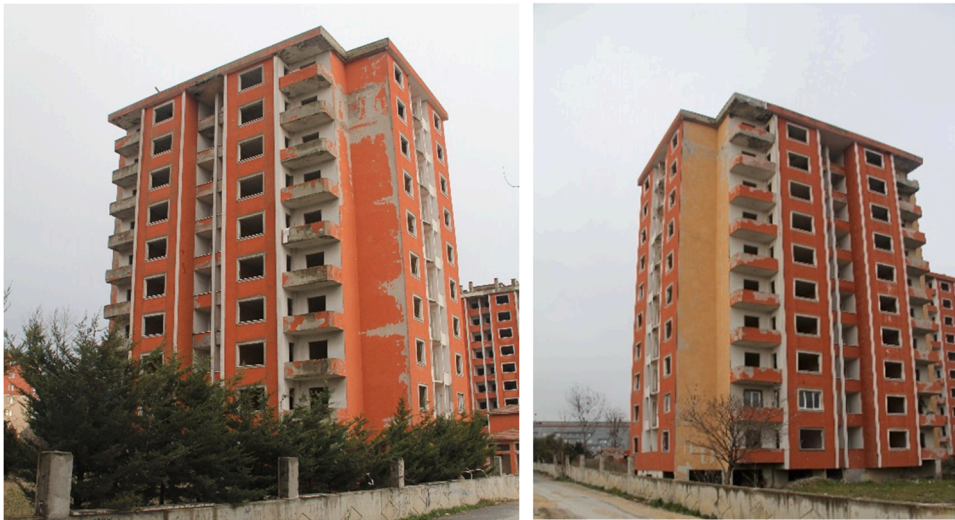
Fig. 2. Overview of Building A.
