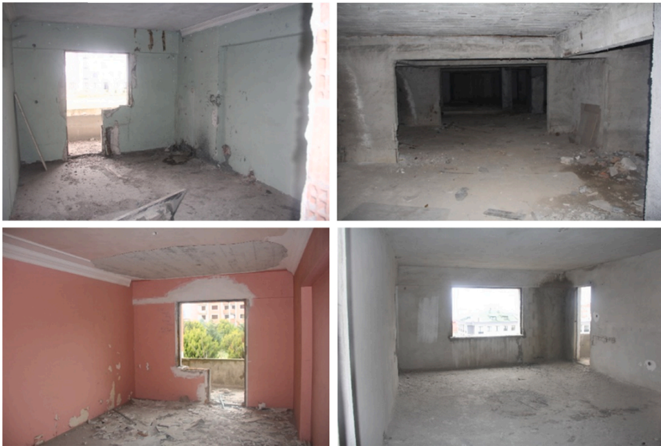
Fig. 7. Interior views from Building C.
