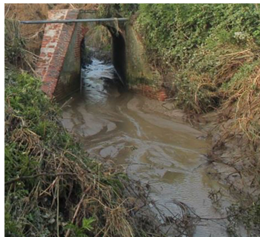
Figure 10. Sarılar village culvert appearance at km: 161 + 955 [21].
