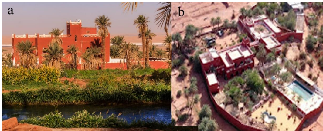
Figure 13 New touristic buildings in old Ksar of Timimoun, (a) Side View (b) Top view.
