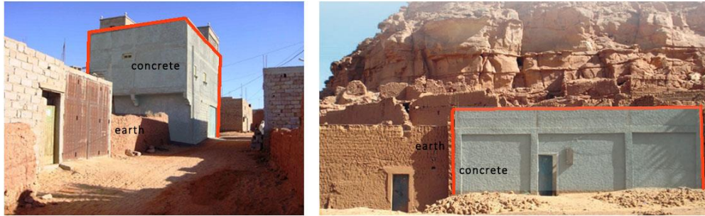
Figure 9 An example for the usage of new construction materials in Ksar (Produced from Rouani, 2017).
