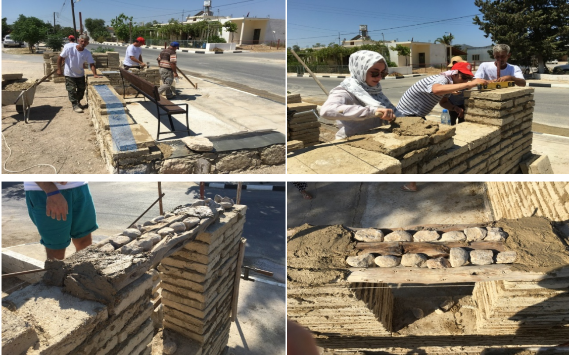
Figure 6. Adobe wall construction, forming of window opening, lintel installation
