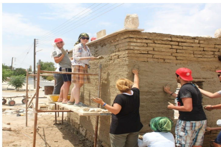
Figure 9. Wall plastering
