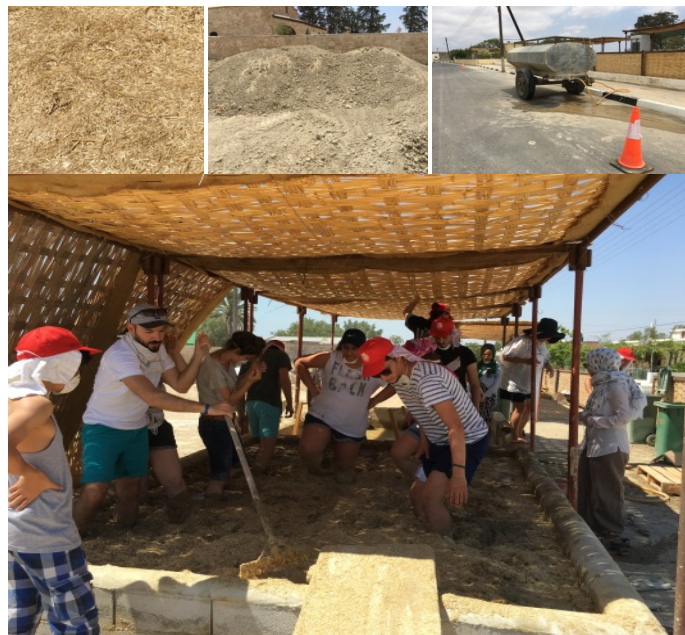
Figure 3. Adobe work area and material content (soil, straw, water)
